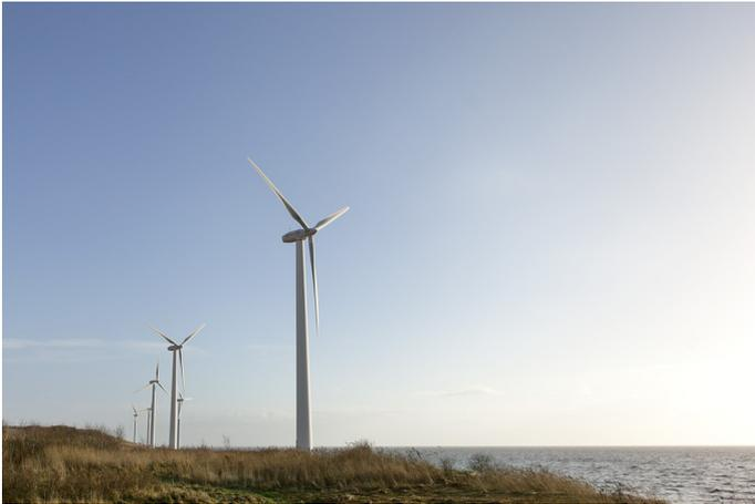
Wind turbines work by pooling the mechanical energy of wind and transforming it into electricity. Wind turns the blades, which spin a shaft, which then connects to a generator and produces electricity. Wind turbines can be built on land or offshore in large bodies of water like oceans and lakes.
